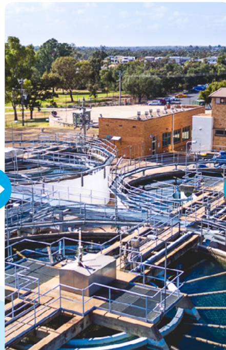
Water treatment Town treatment plant
