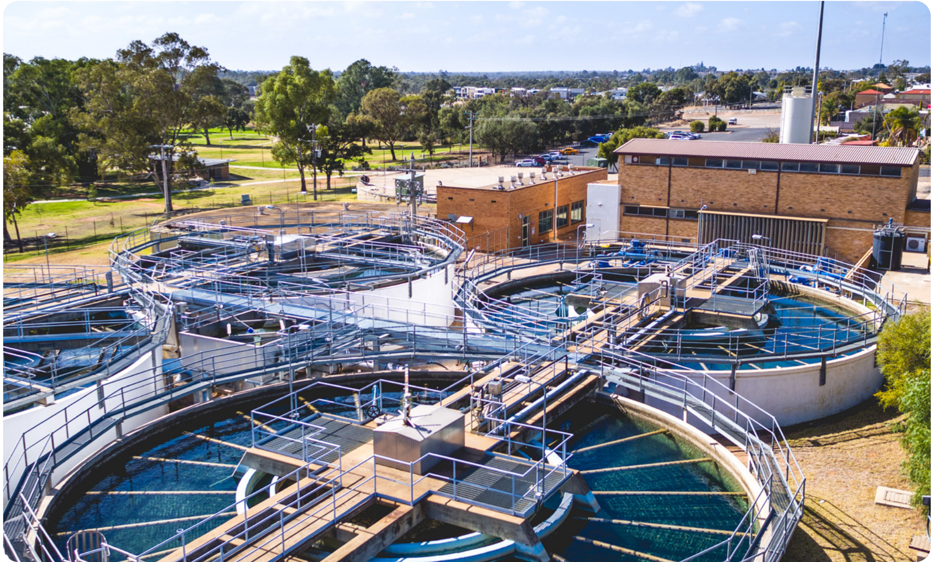
Water treatment plant, Mildura
