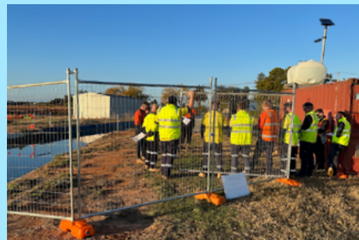
Site inductions at Red Cliffs Channel.
